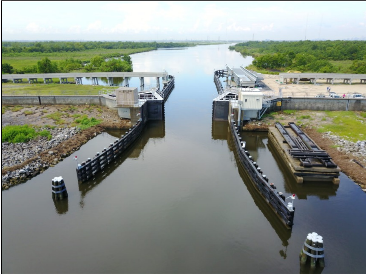
Figure A-95: Example Sector Gate (HSDRRS, Bayou Bienvenue Gate at Back Levee)
