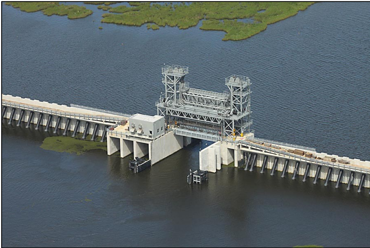
Figure A-84: Example Vertical Lift Gate (HSDRRS, Bayou Bienvenue Gate at Surge Barrier)
