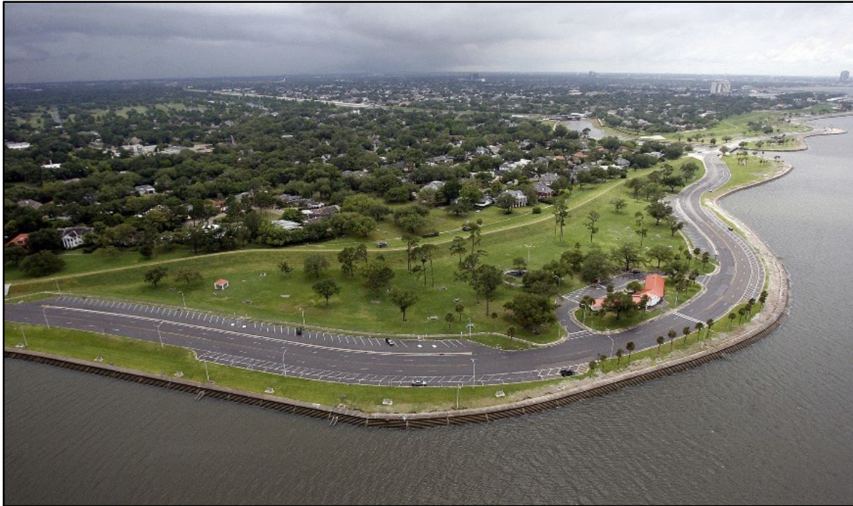
Figure 4-15: Lakeshore Drive, New Orleans, with Seawall and Levee System (Michael DeMocker/NOLA.com | The Times-Picayune )
